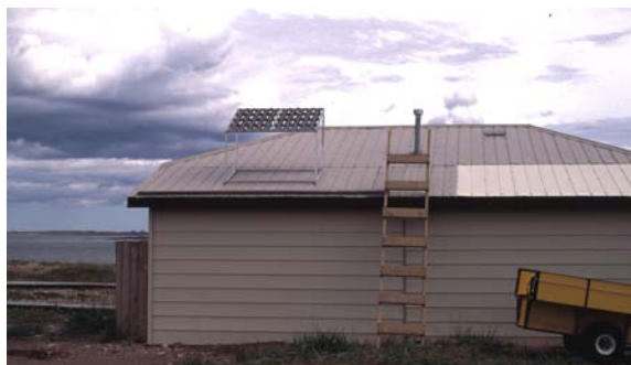
Figure 2: Coupon rack installed on roof of modern building.
