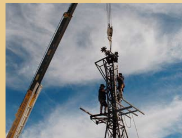
Head of the mill lifts off after being in place for close to 90 years.
