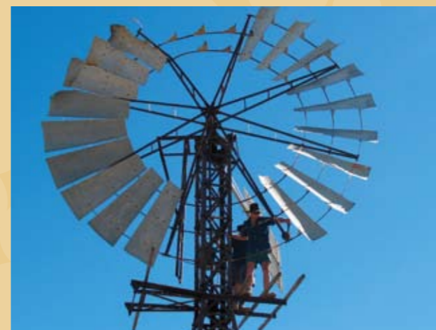
Removing the fans. Note that the removal is done maintaining the balance of the wheel as much as is possible.
