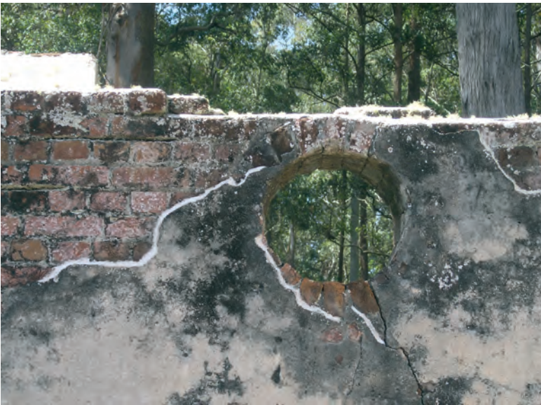
Holes in the exterior walls of the Lake Innes House stables allowed owls to fly in to catch rats and mice.
