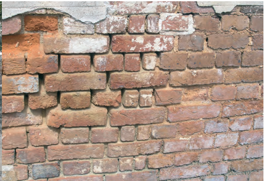
Bricks made by convict labour from clay on the Lake Innes Estate, and baked in ovens on site.
