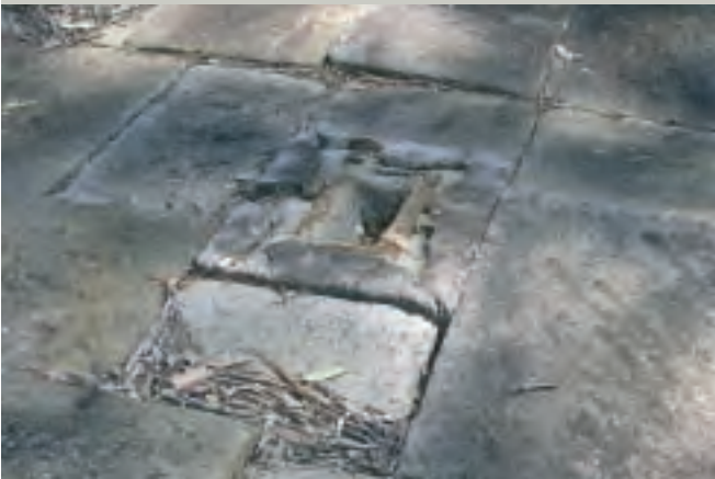
Dressed stone flags in the stables at Lake Innes House show the attention to detail lavished on their construction.
