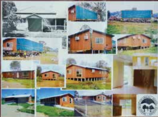
Top Left: Original Brungle Station Managers house. Others: Brungle Health Centre building, 2005.
