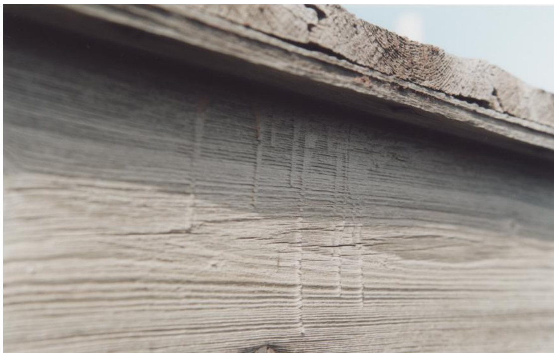
Figure 7: Early wood has been removed by wind ablation on Discovery Hut leaving late wood in pronounced ridges. Note paint drip lines afforded longer protection leaving a last vestige of the original surface.
