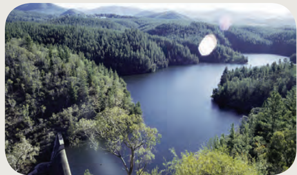
Cotter Dam in the 1990s. This dam, Canberra's oldest, will soon be drowned by the Enlarged Cotter Dam, being built to protect Canberra's water supply against drought induced by climate change.
